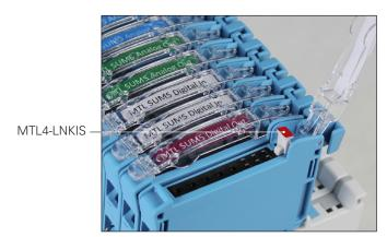
Link LK1, referred to in the safety parameter specification and shown on the module schematic, is the MTL4-LNKIS link and is primarily used to increase the output power from the MTL4-ADIO when being used in Digital Output mode with solenoid valves. If the valves are suitably certified this link may be fitted to increase the available power and voltage to the valve. It may also be used for analogue input and analogue output applications, if required, where the field device is suitably certified.
